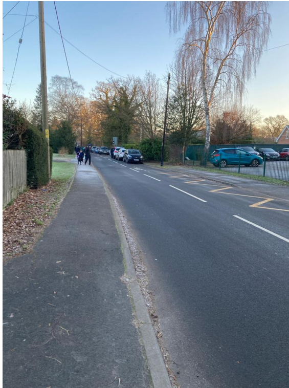
Image 7: School Road, North of entrance to School, looking towards A321. 11 January, 2024 @ 08.37
